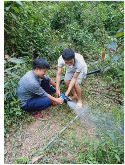
Figure 16. water pipe system installation for 59 households with limited water access
